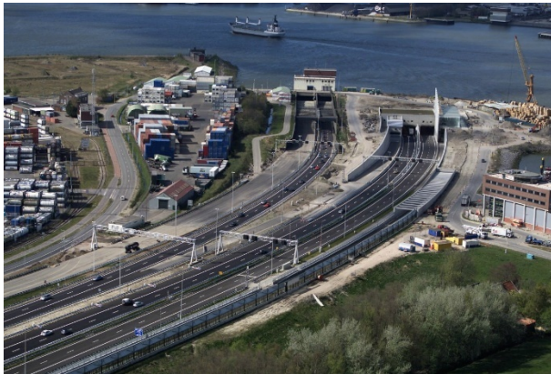
(c) Second Benelux Tunnel, Rotterdam
