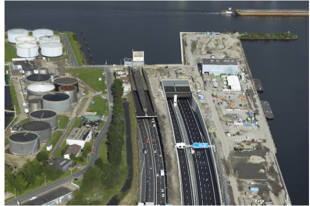
(b) Second Coen Tunnel, Amsterdam, The Netherlands
