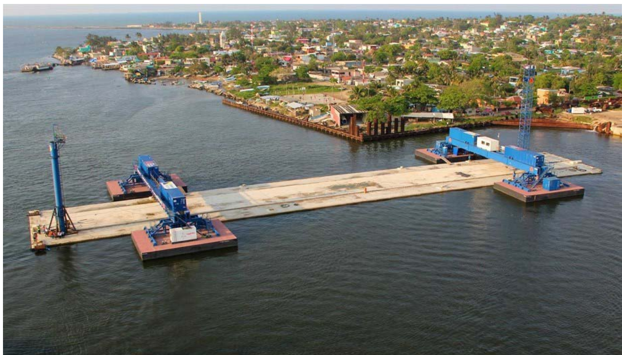
Figure AA Coatzacoalcos Tunnel in Mexico being placed in the River Coatzacoalcos 59 .
