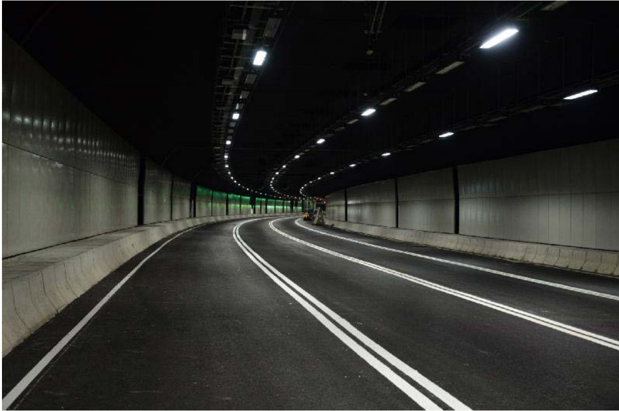
Figure HH View inside a completed tunnel tube with three driving lanes and a shoulder for the Hong Kong Zhuhai Macao Link in China 64 .
