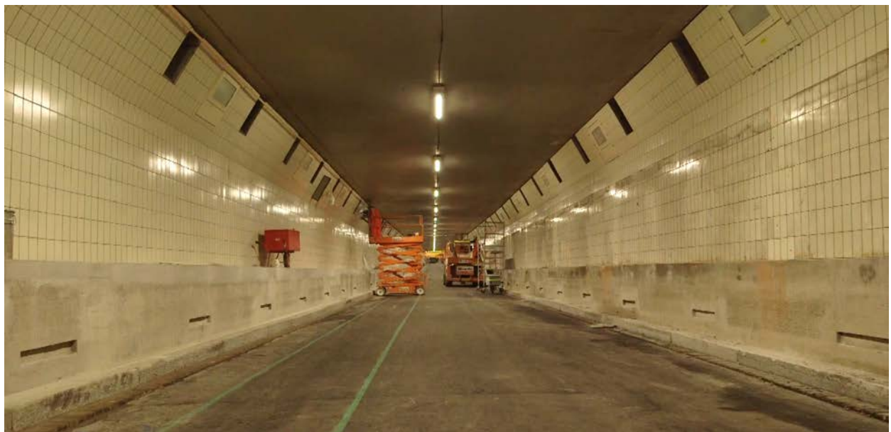
Figure Y Retrofitting of the Maastunnel currently underway 55 .
