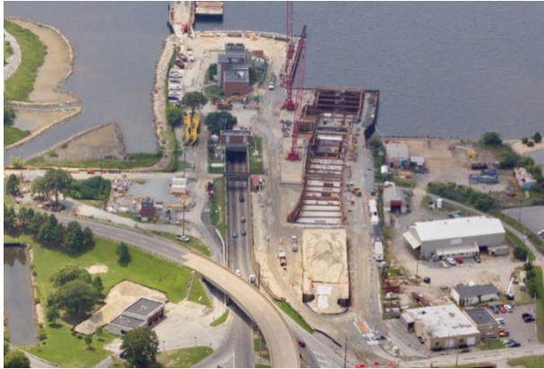
(a) Elizabeth River Tunnels, Norfolk, USA
