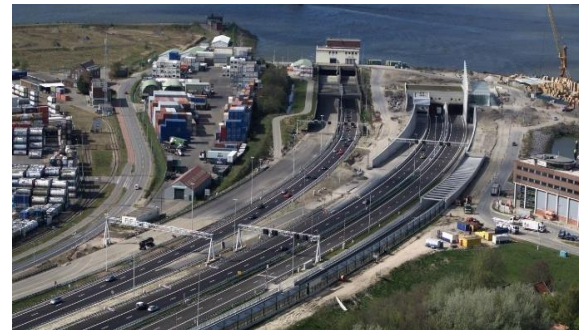
Second new ITT constructed next to existing older ITT in Rotterdam, Netherlands. (below)
