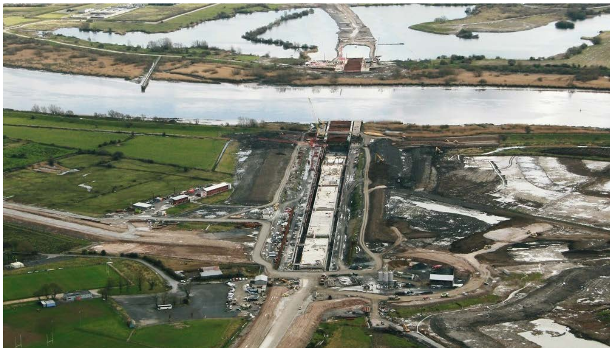
Figure CC Tunnel elements being fabricated in approach to ITT crossing 61 .
