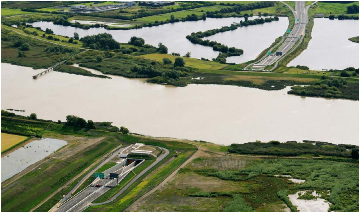
Figure BB Limerick Tunnel located under the River Shannon near Limerick, Ireland 60 .
