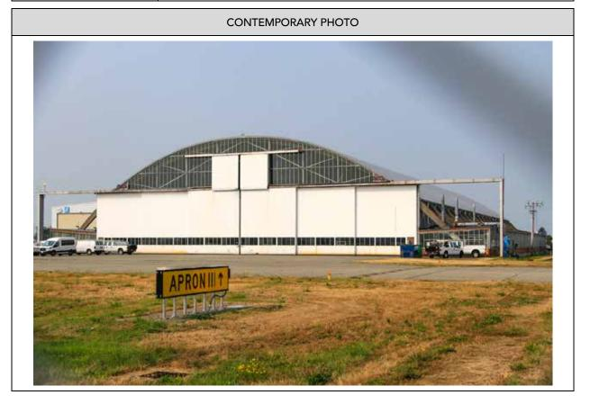
The Britannia Hangar is a large aircraft maintenance facility built for Canadian Pacific Airlines in 1958 and located in the South Terminal area of the Vancouver International Airport. Featuring an arched roof and structural concrete arches, the unique design of the hangar provides ample, uninterrupted space for aircraft service.
