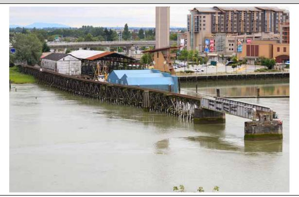
The Vancouver and Lulu Island Railway Bridge extends part way into the North Arm of the Fraser River, originally connecting Vancouver and Richmond's Lulu Island. The bridge is characterized by its solid timber trestle structure.
