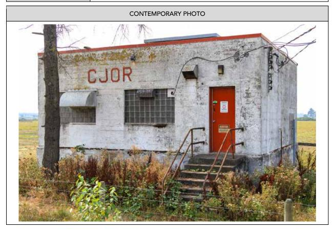
The CJOR Transmitter Station is a small rectangular concrete building located along Nelson Road in an agricultural area of East Richmond. The modest building is characterized by its board-formed concrete construction, flat roof, and glass block windows.
