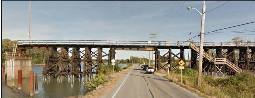
The existing maximum road clearance below the structure is posted at 5.88 m. Raising the road/dike would reduce the clearance.
