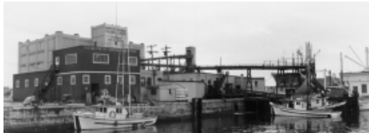
The photo on the right, from the BC Packers Insurance Series, shows Victoria Cold Storage Plant in 1961.
