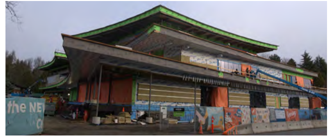
Steveston Community Centre and Library Construction
