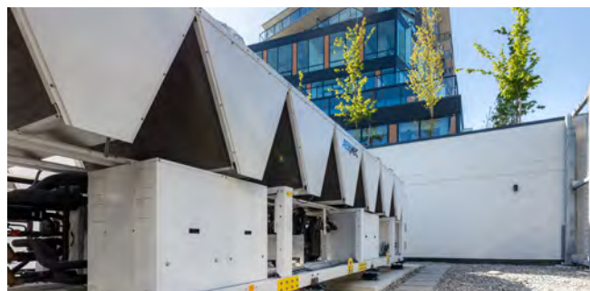
CCDEU Expansion Project
