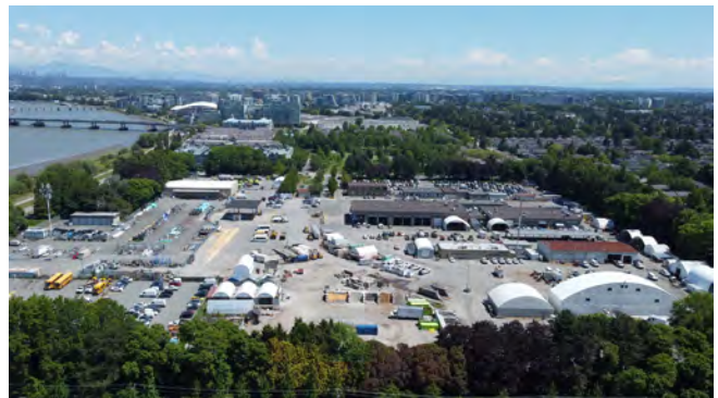
Major Construction Project – Works Yard Replacement Project
