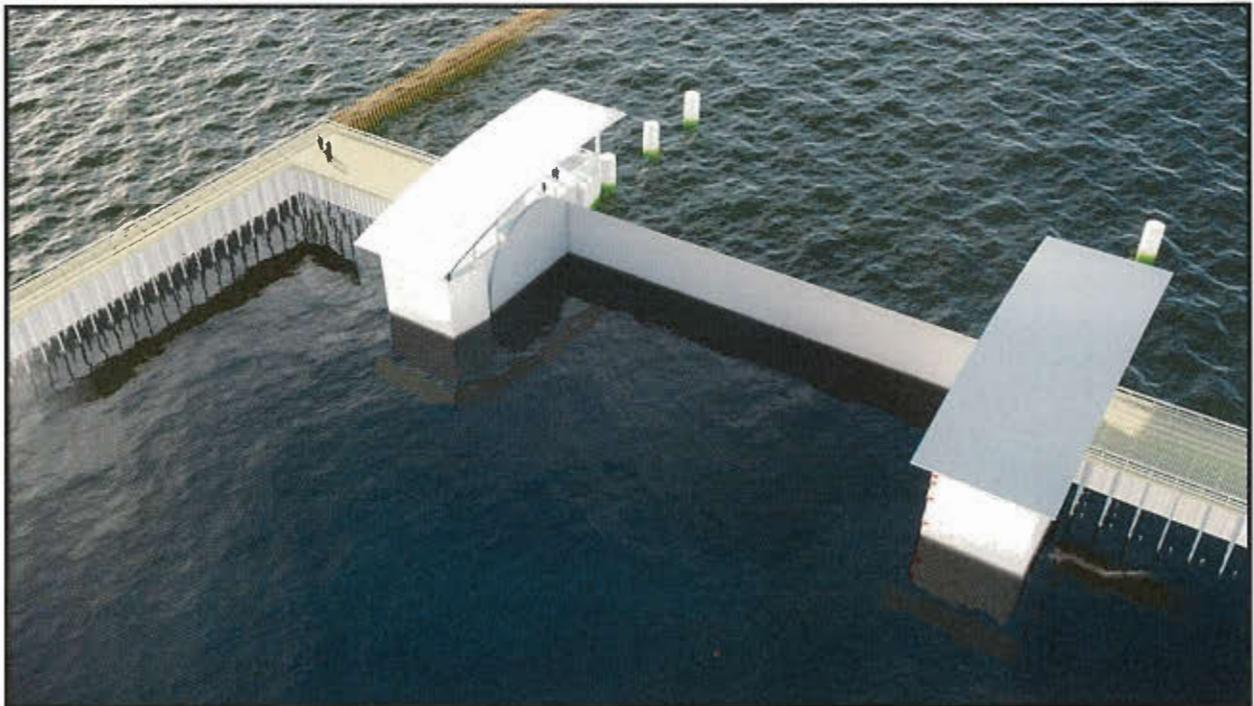
Figure 3. Closed Horizontal Axis Sector Gate (Looking West) Rendering
