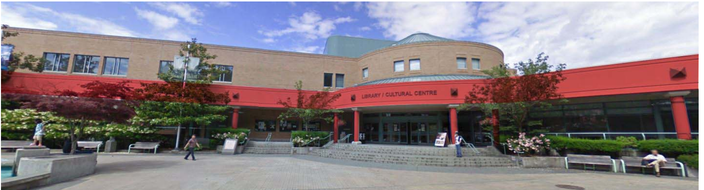
Figure 2 – Exterior fascia banding and columns, highlighted in red at Cultural Centre Plaza entrance.
