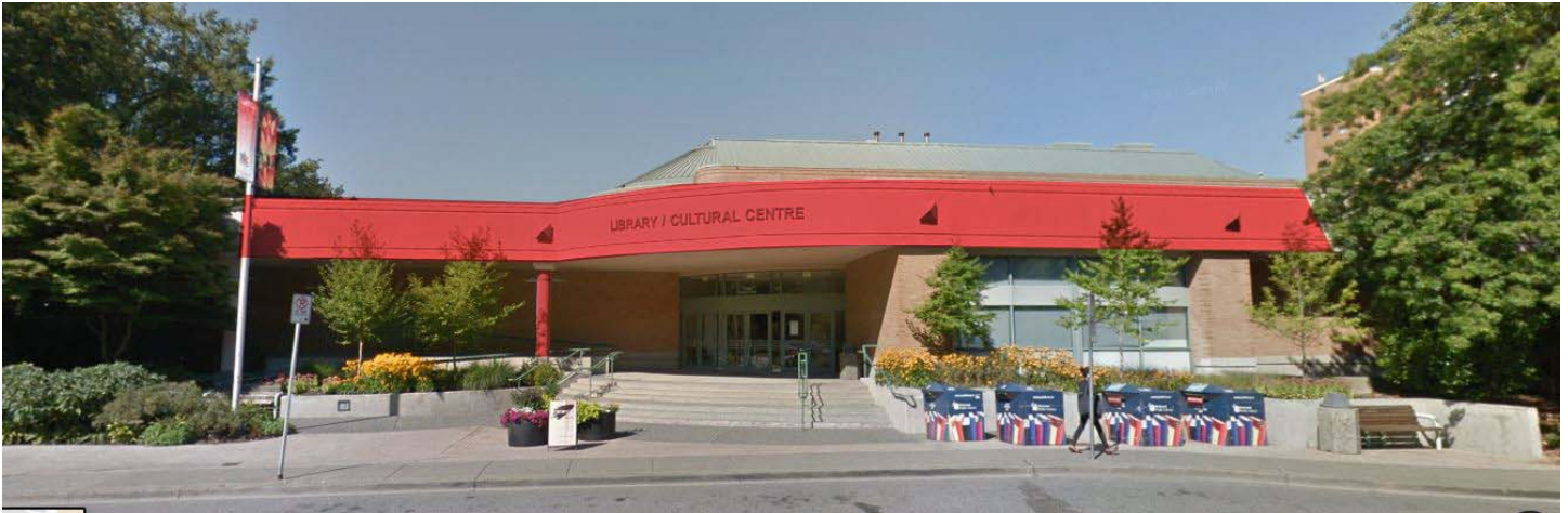
Figure 1 – Exterior fascia banding and columns, highlighted in red at Minoru Gate entrance.
