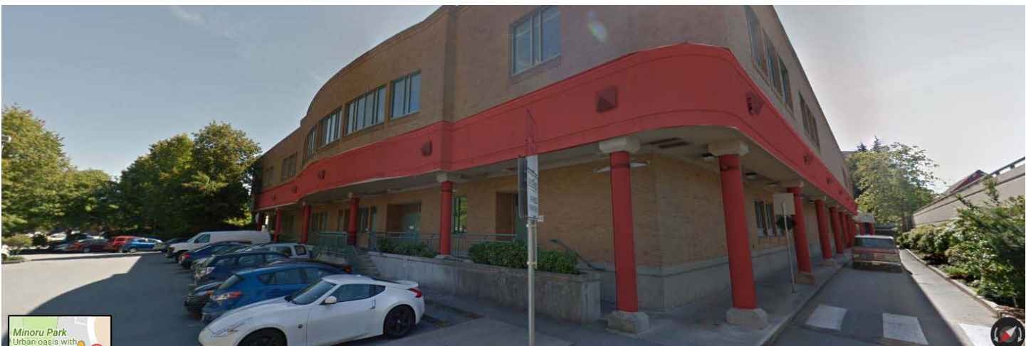
Figure 3 – Exterior fascia banding and columns, highlighted in red at north parking lot and east access lane.
