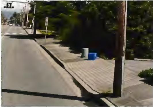
Figure 1: Before - Older Design with Utility Strip and 1.5m Sidewalk
