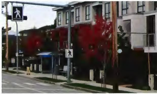
Figure 2: After - Current Design with Boulevard/Utility Strip and 1.5m Sidewalk
