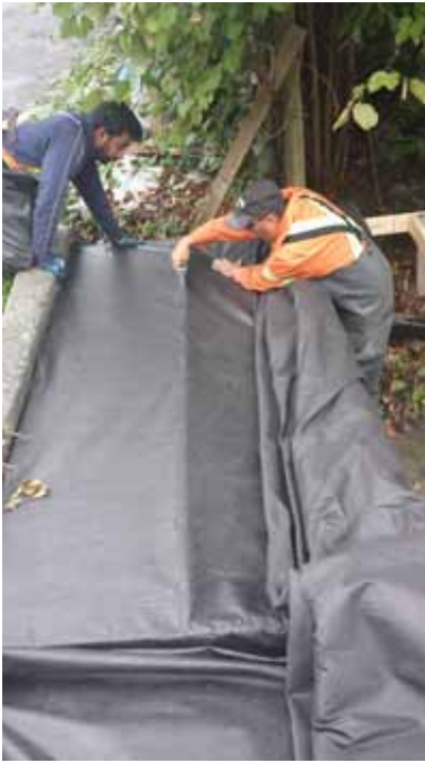
City crews place a shading frame over a ditch to discourage growth of Parrot's feather, a sun-loving aquatic weed
