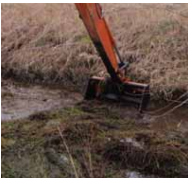
City crews apply best management practices for parrot's feather control, while maintaining a City watercourse
