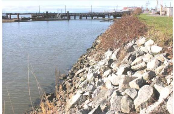
constructed or upgraded during the Fraser River Flood Control Program. Upgrades to the dikes in Steveston took place in the late 1970's. At that time, the dikes were generally upgraded with expansions to the land side and increases to crest height and width.
