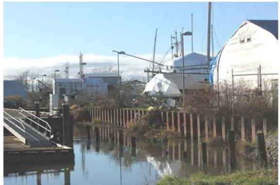
A floodwall can be constructed from a number of different materials including concrete, steel or plastic. Some floodwalls can be designed to be demountable and are only erected prior to a flood. There are some existing examples of sheet pile floodwalls in the Steveston Area.
