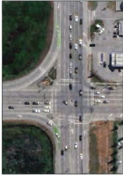
Figure 12: Intersection of Westminster Hwy and No. 5 Road (Source: Google Earth)
