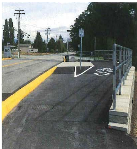
Figure 2: Bike Lane Treatment at Bus Stop on Westminster Hwy
