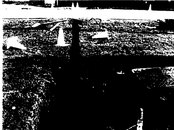
Vactor Trucks are used to suck soil from neat trenches leaving tree roots and existing utilities intact – note little disturbance to surroundings and roadway.
