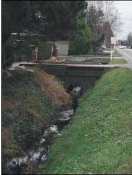
Open ditches along Blundell Road
