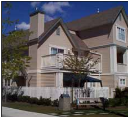
Porches and Balconies
