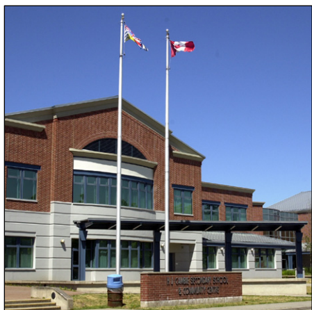
Cambie Community Centre and School
