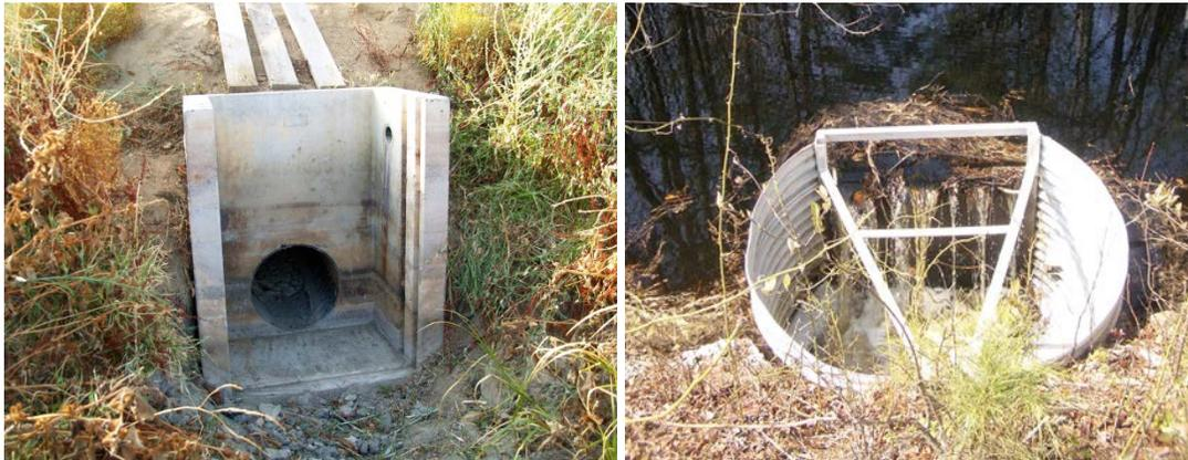
**Figure 10-4: Examples of the Wetland Outlet Structures**
