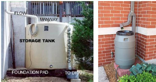
**Figure 12-1: Example of Rain Barrel and Cistern**
