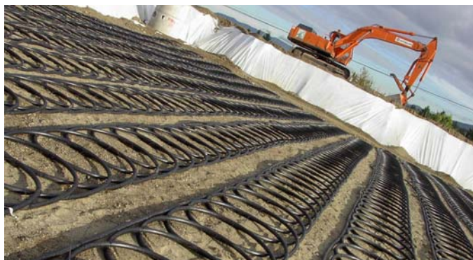
GeoTility installed the largest horizontal heat exchanger in Canada at the headquarters of Tekmar Control Systems in Vernon, BC, 2003. Photo credit: GeoTility Archives.
