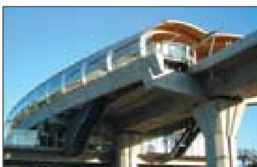
10. Transit Station at its Centre
