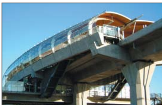
10. Transit Station at its Centre
