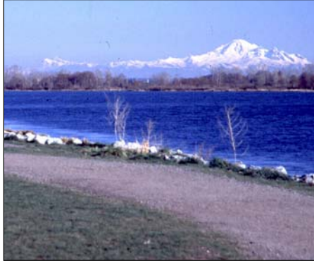
Richmond's dyke system provides floodproofing protection
