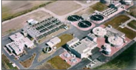
Lulu Island Sewage Treatment Plant
