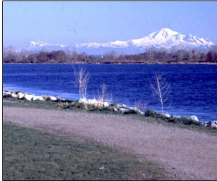
Richmond's dyke system provides floodproofing protection
