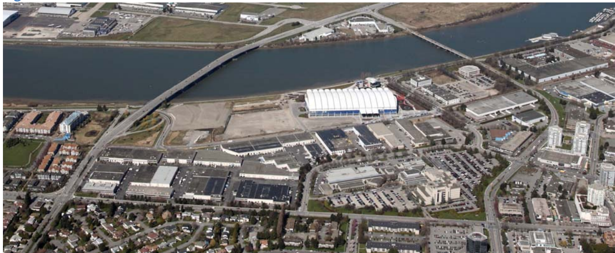
Figure 1: River Green – Aerial
