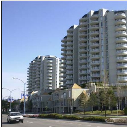
Townhouses at street level
