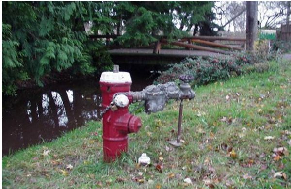
Figure 9: Backflow Prevention Device
