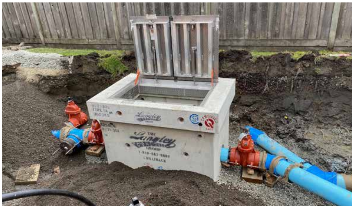
Multi-Family Water Meter Installation
