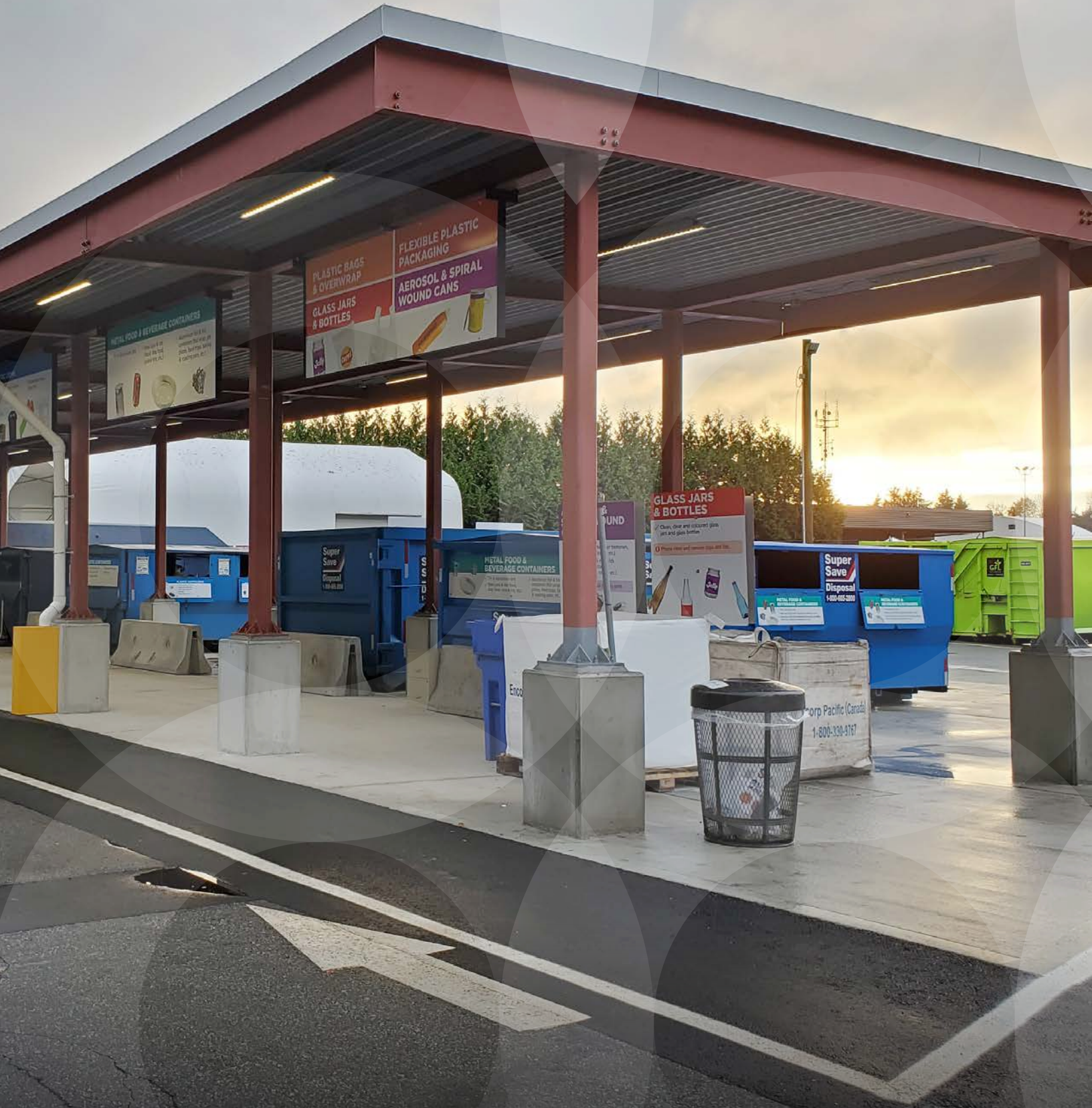
RENOVATED IN 2020, THE RECYCLING DEPOT UPGRADE IMPROVED CONVENIENCE AND BROADENED THE SCOPE OF SERVICES FOR RICHMOND RESIDENTS.
