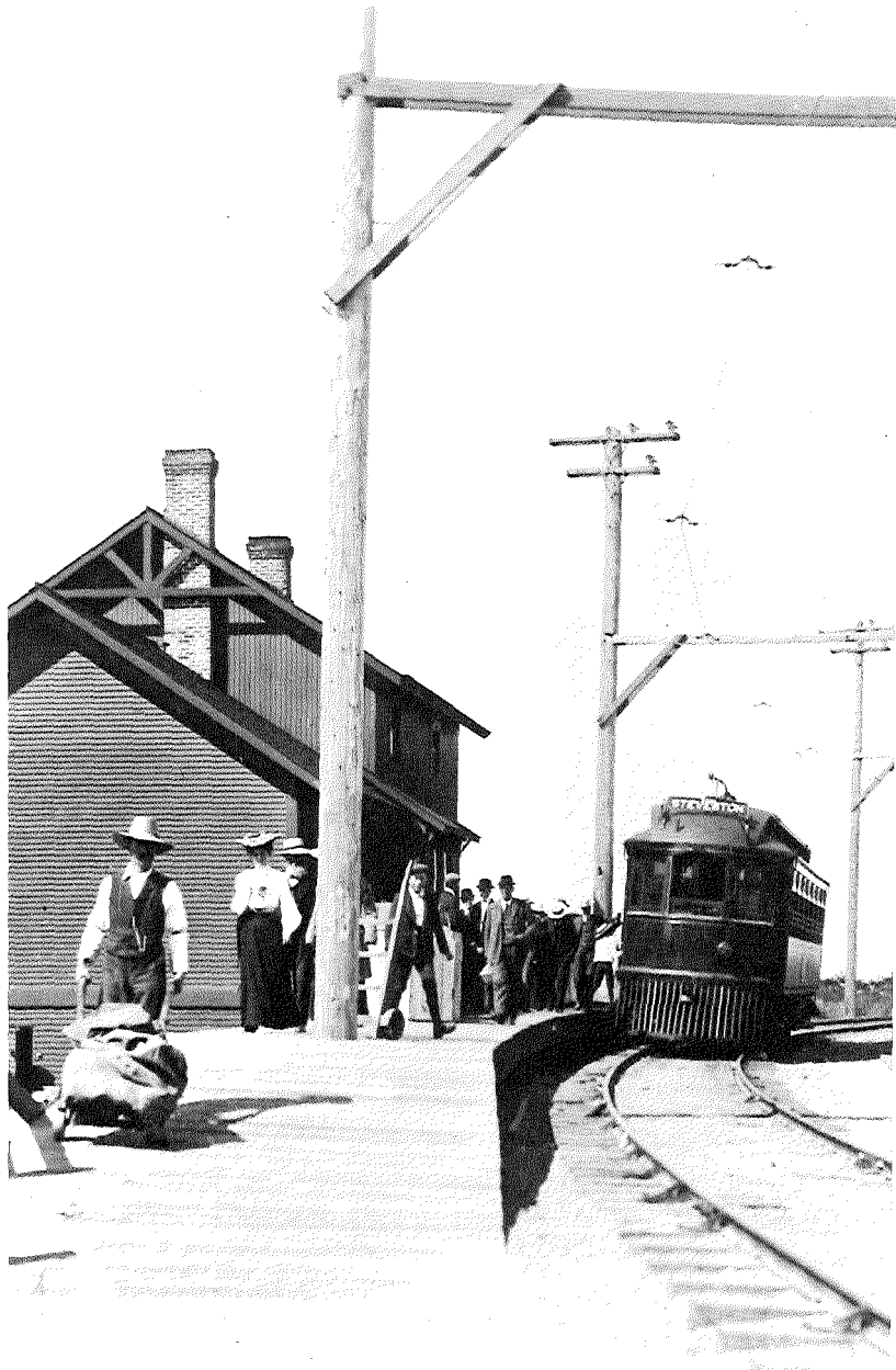
58. B.C.E.R. tram bound for Steveston, c.1908.
