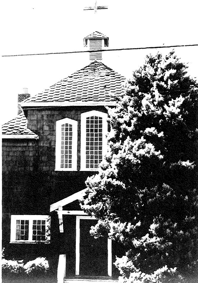
258. A rear view of St. Anne's Anglican Church, Steveston.
