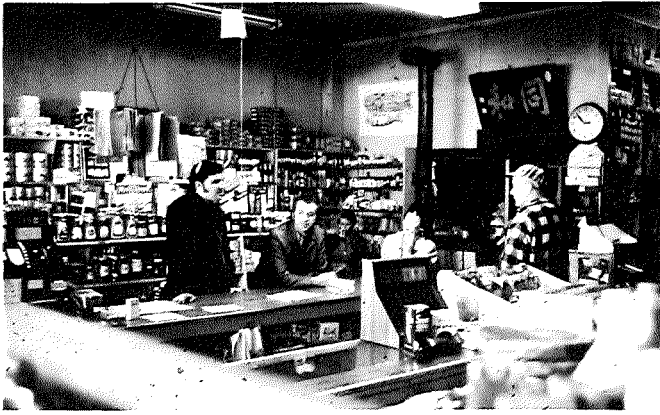
226 .The well known Hong Wo "living in harmony" store on the dyke near Steveston. The store and adjacent buildings were burned down in the summer of 1977.
