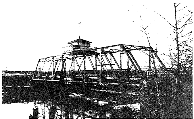
286. Fraser Street Bridge.
