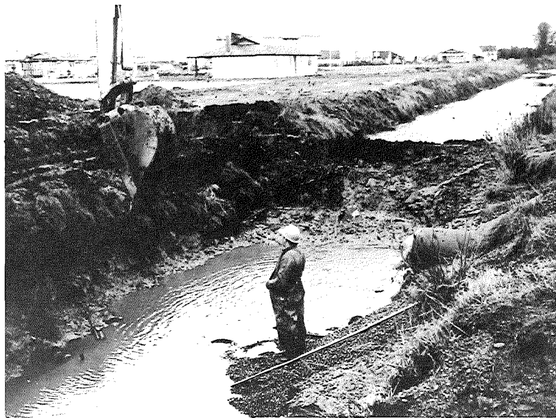
338. Dredging ditches for new canals.
