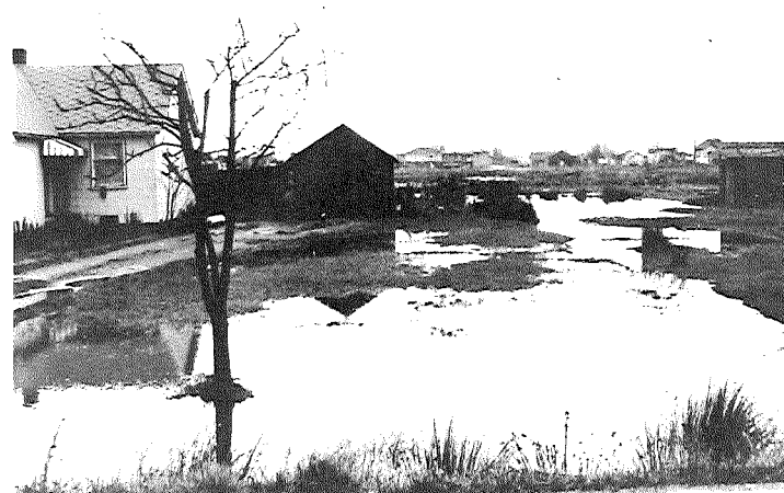
336. Aftermath of heavy winter rains.
