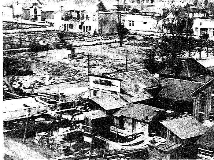
137. Overlooking Steveston after the fire of 1918. The street crossing the page is Moncton Street. On the south side of the street standing alone is the Hepworth (Brick) Block.
