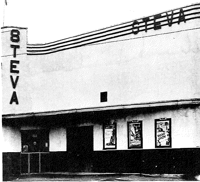
309. The Steva Theatre, Steveston, opened 1947.
