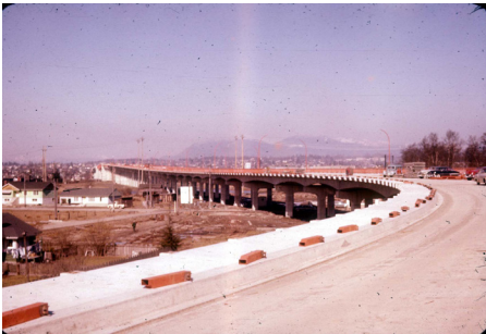
Oak Street Bridge construction, March 1957, 1957. Bill Topping fonds. City of Richmond Archives, photograph #2008 36 2 23.
